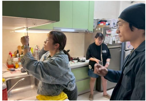
04/12 桃區【水電維修】安裝燈條
